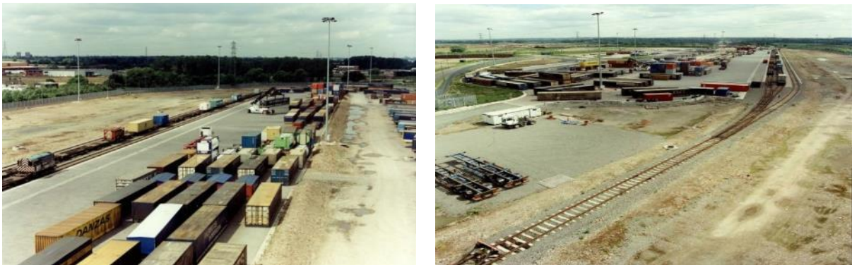
Figure 10 Hams Hall Phase 1 handling area
