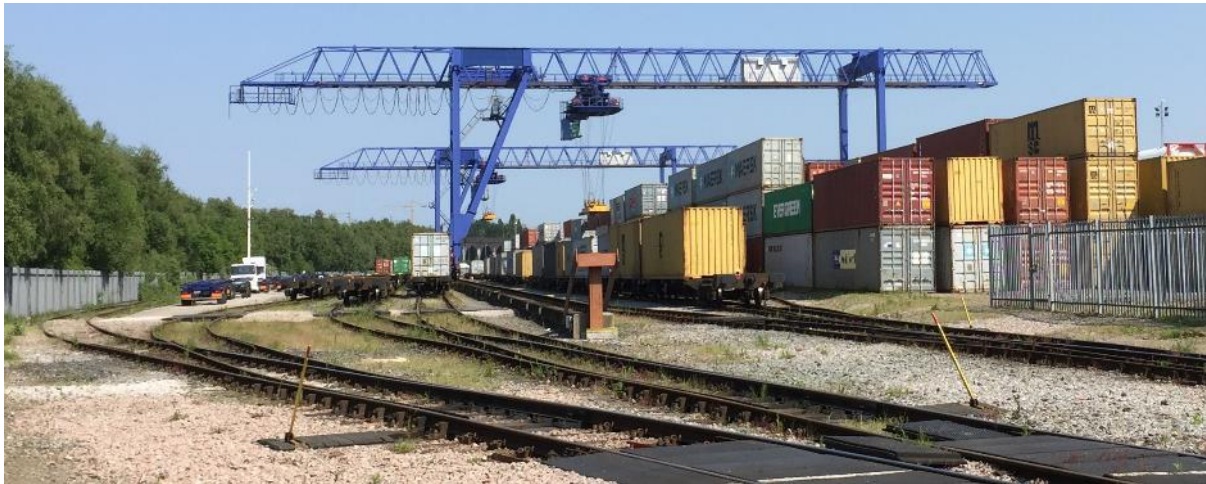
Figure 5 Rail sidings and container stacking area, 3MG Widnes
